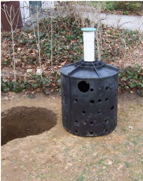
ROCK INFILTRATION CHAMBER - DOWNSPOUT CONNECTION
